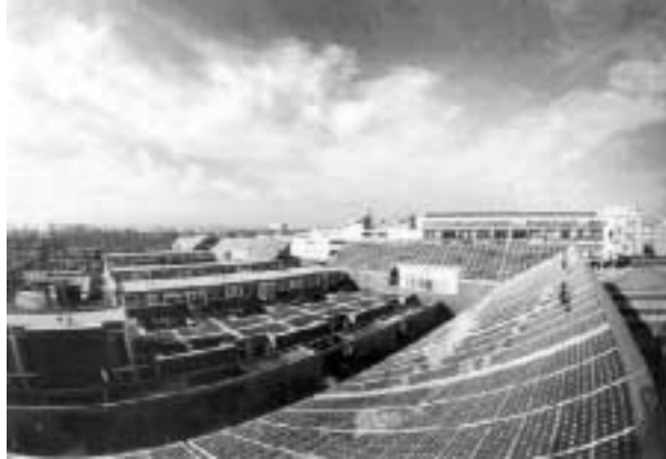
Fig 10. Wide-angle shot of the Nieuw Sloten project. In the front the roof facing west, in the background the apartment building with PV facade and the two penthouses. To the left the shaded east roof can hardly be distinguished.
