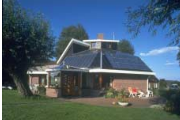
Fig 4. The zero-energy house Woubrugge, first project in the Netherlands with PV as watertight roof cover.
