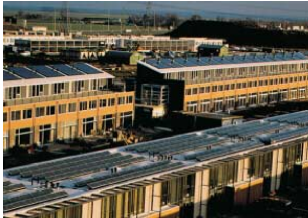
Fig 11. The PV project Nieuwland during installation.
