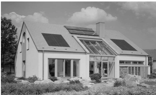
Photo 5: Example of "Braas Solar Roof Tile", 1,4kWp, Alzenau
