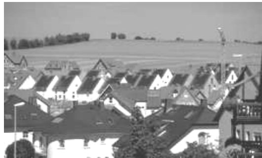
Photo 8: PV-Roof integration, 72,6kW p , "Sonnensiedlung", Hettstadt
