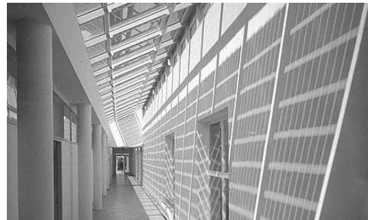
Photo 6: PV-Rooflight, 4,0kWp, Local Utility, Halle
