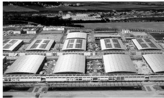
Photo 10: PV-Roof integration, 1.16MWp, New Trade Fair, Munich
