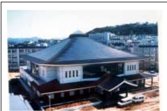
Fig. 2: Japan. Houoh High School. NEDO commercial roofing tiles
