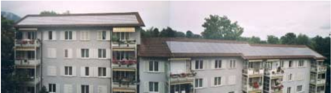
Fig. 2: 53.04 kW PV installation ABZ for the 'Solarstrom stock exchange' with SOLRIF (in this figure only one house row, 26.52 kW is shown)
