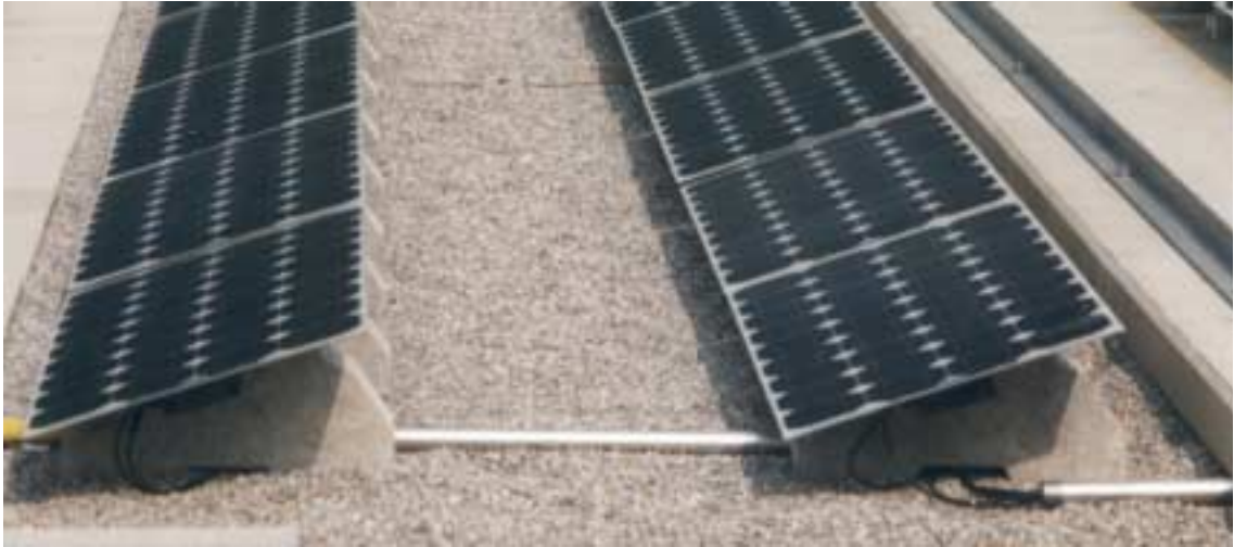
Fig. 3: Most commonly applied mounting structure for flat roof installation within the 'Solarstrom stock exchange'.
