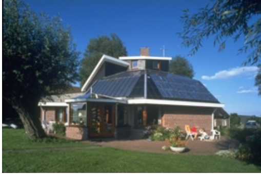
Fig. 5. The zero-energy house Woubrugge, first project in the Netherlands with pv as watertight roof cover.
