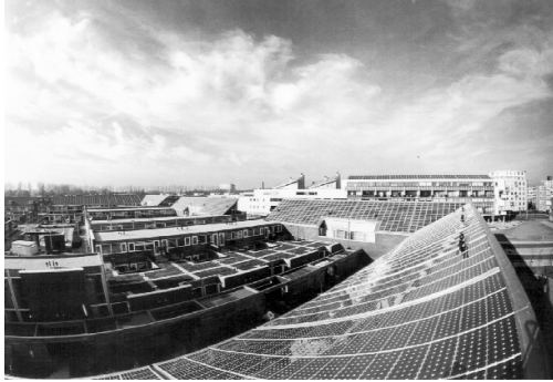
Fig. 10. Wide-angle shot of the Nieuw Sloten project. In the front the roof facing west, in the background the apartment building with pv facade and the two penthouses. To the left the shaded east roof can hardly be distinguished.
