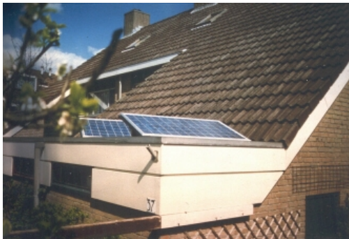
Fig. 9. Two AC-modules on the roof of a private residence. A new market for pv.
