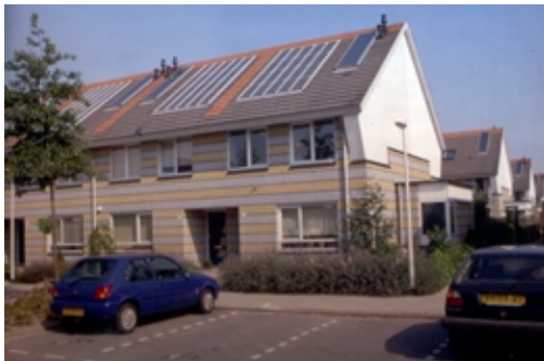
Fig. 8. Barendrecht. The first project in the Netherlands featuring building integrated pv on a commercial basis.
