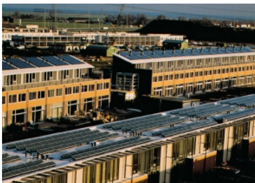
Fig. 11. The pv project Nieuwland during installation
